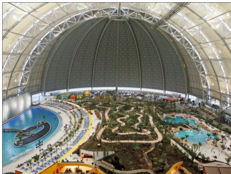
Examples of structural domes in Water Parks. Source Internet :Aircrafw
